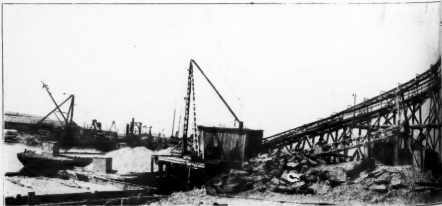
The Long Beach Plant Showing the
